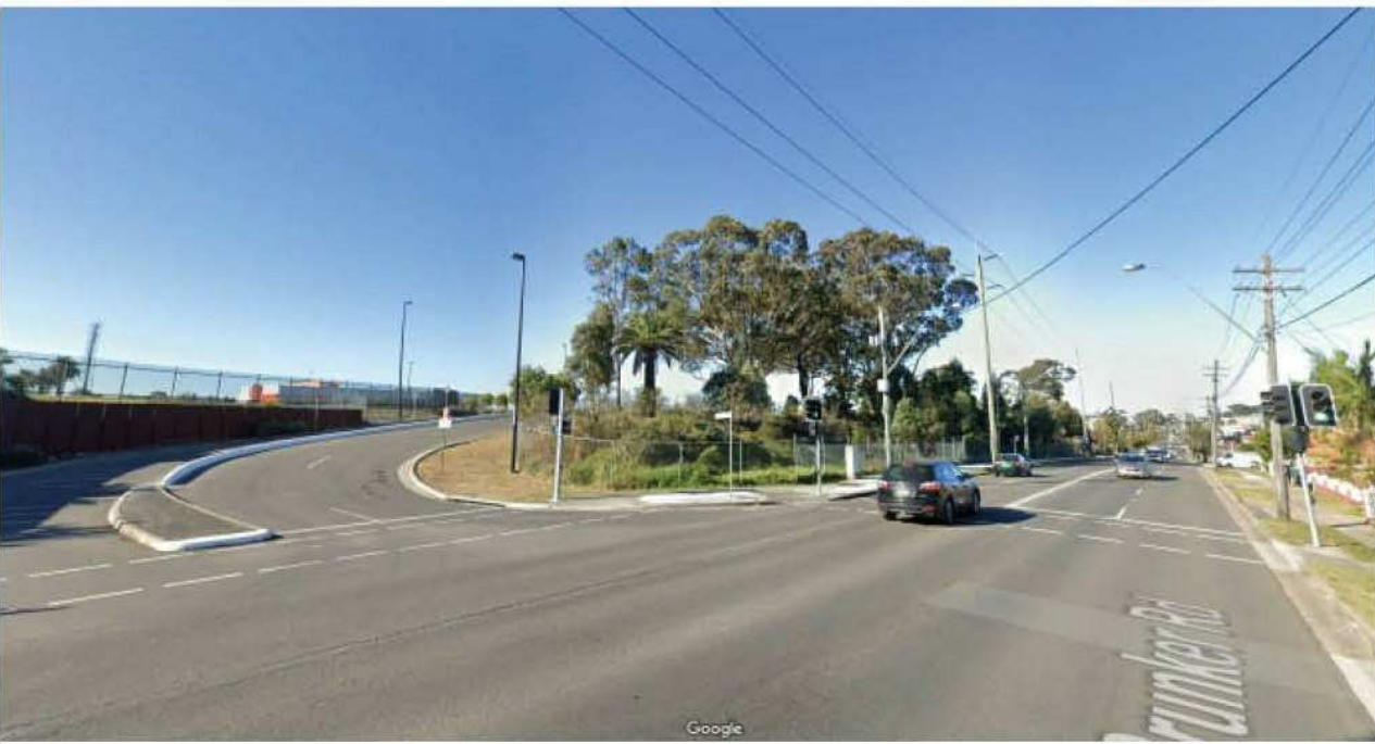
NELSON SHORT ST WITH BRUNKER RD
